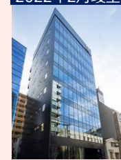
S-GATE FIT 八丁堀
